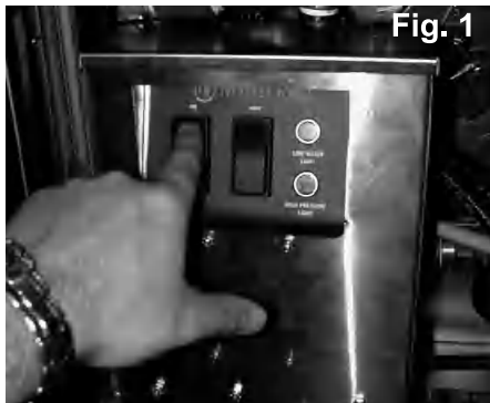
1. Energize boiler and fill to operating level.
